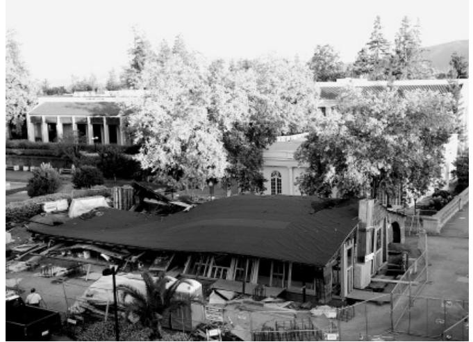
Cottage collapse. Photo by Rodney Fernandez, 6/02/2010.
